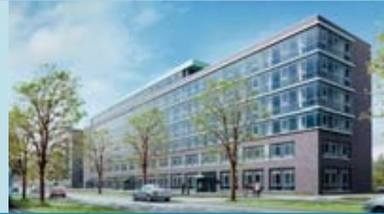
Presently, the Bauwo Business Center is being built along Hans-Böckler- Allee as part of phase three. This is an office and admin building of approx. 10,000 sqm.
