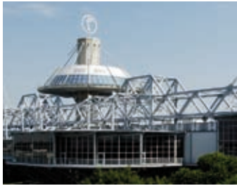
Outside view of the Convention Center
