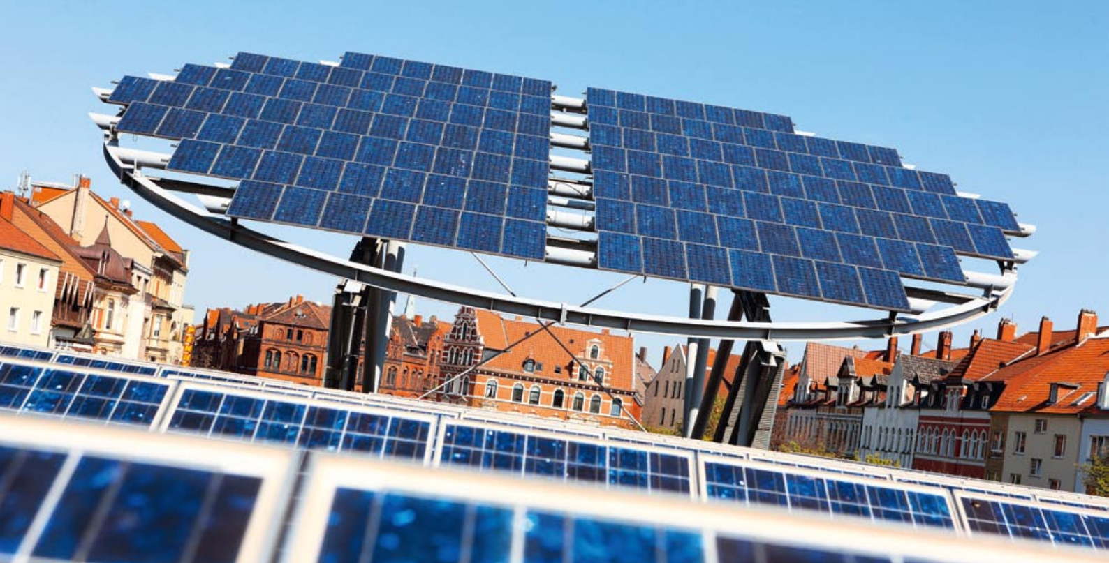
Solar panels mounted on the roof of the Pavillon cultural centre
