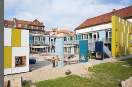
Right: Passive-house construction of children's daycare centre in Ricklinger Strasse
