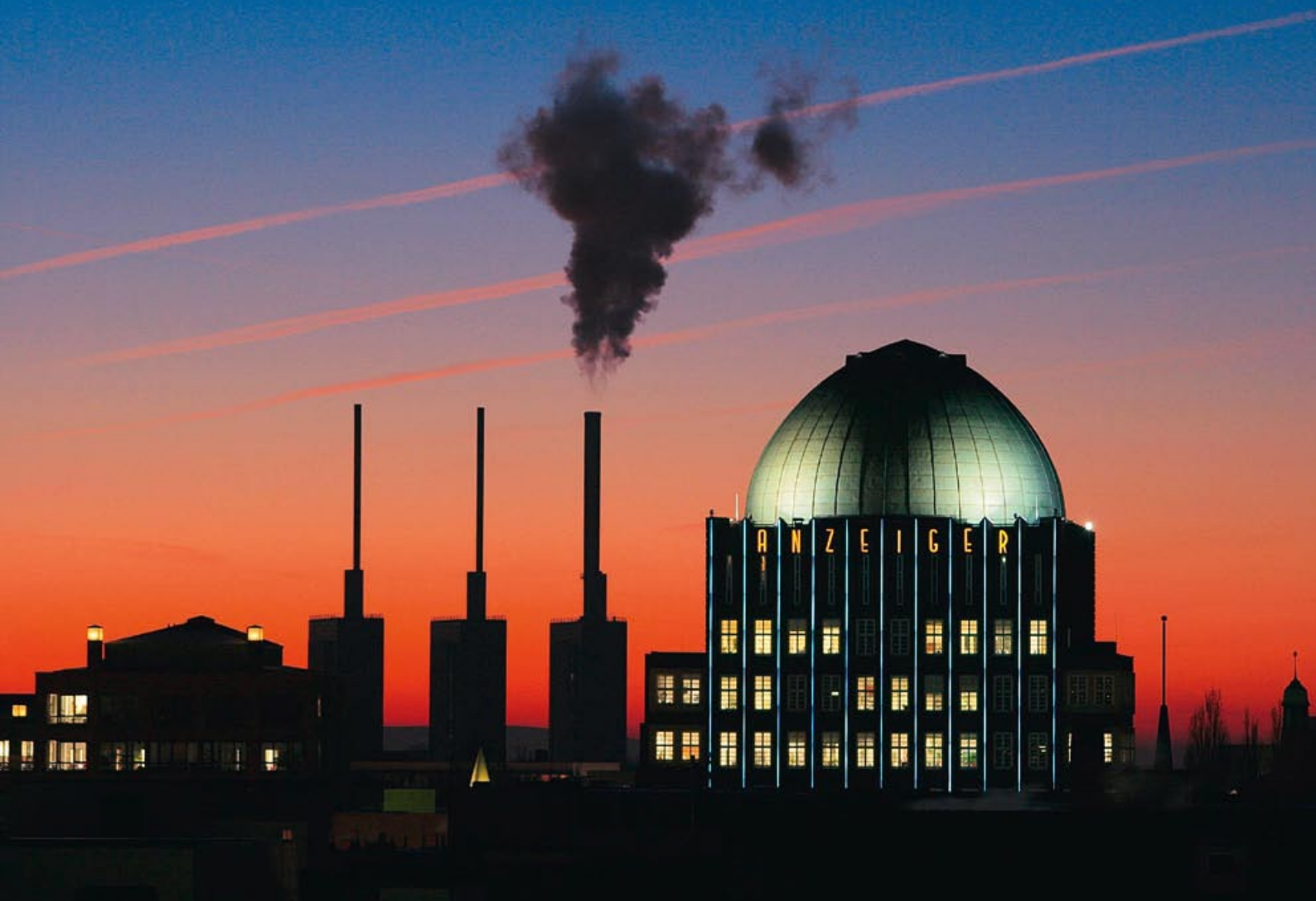
Linden power station with gas and steam turbines. In the foreground is the Anzeiger building, which belongs to the Madsack publishing company
