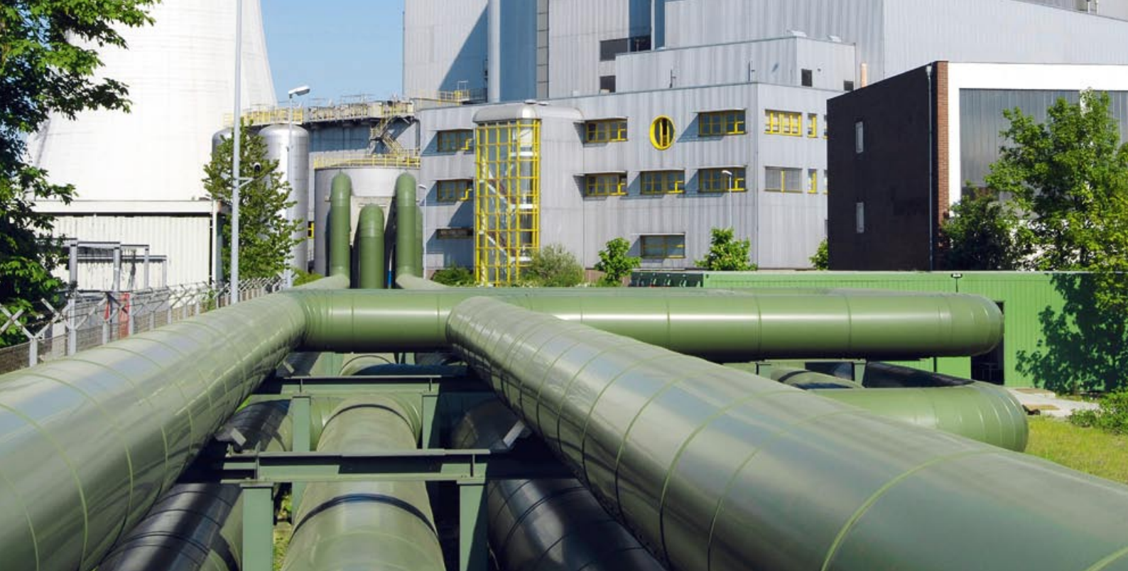
Top: District heating pipelines at the power station in Hannover-Stöcken Left: CHP unit in Ostwender Strasse Right: CHP unit of the sports club Sportgemeinschaft von 1874 in Hannover-Herrenhausen Far right: CHP unit at the GBH Mieterservice
